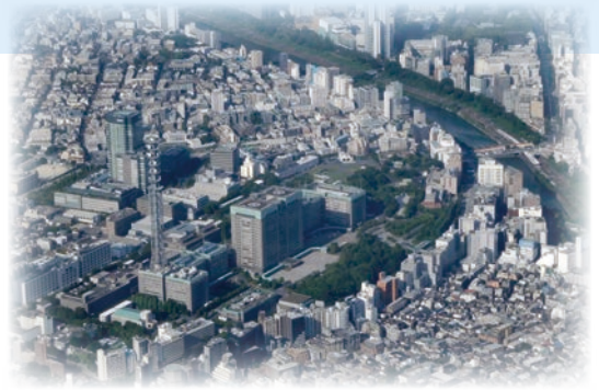
JMOD Head Office of Ichigaya Area
