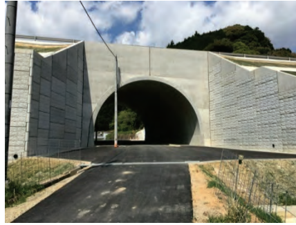
②Max Arch B12.3×H8.81, 施工延長25.5m
